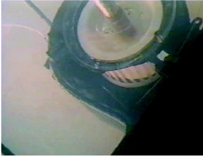
Fig.1 HVAC fan module used in the flow visualization study
